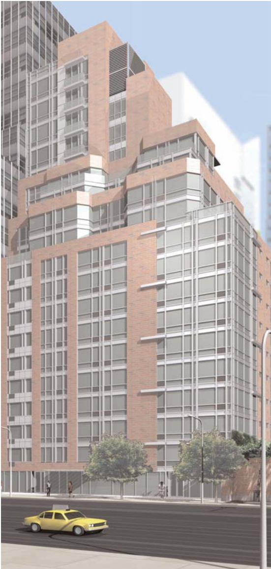
↑ 211 East 51st Street New York, NY Addition of 8 Stories onto an existing 14 story structure. Conversion of entire building to condominiums. Architect: Meltzer Mandl
