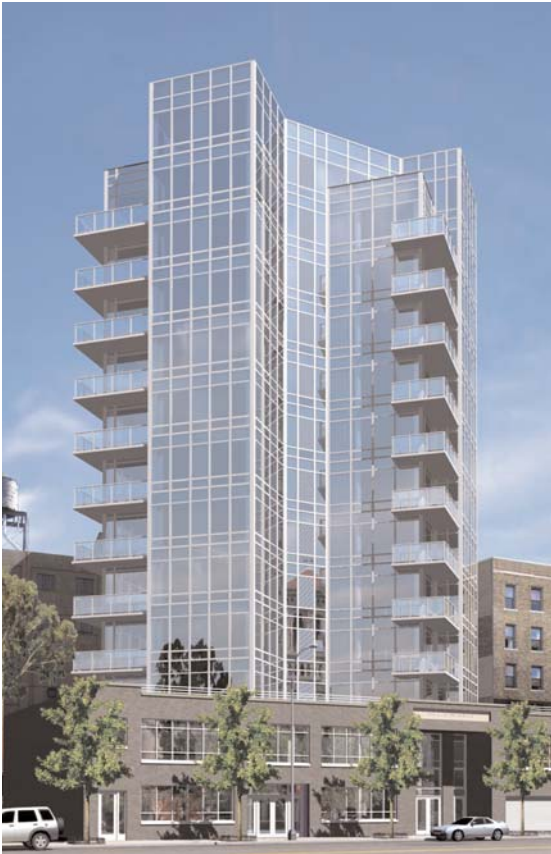
← 525 Clinton Avenue Brooklyn, NY New 12 story all glass curtain wall building, with 30 high end residential condominium units. Each dwelling unit is provided with a separate direct vent boiler and air cooled AC unit. Architect: Simon Fouladian Owner: Clinton Court Development
