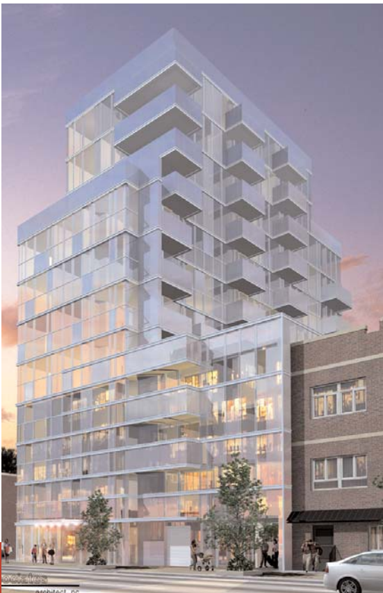
← 202 8th Street Brooklyn, NY 12 story 50,000+ sf high end condominium, with outdoor eating areas and glass facade. Architect: DJ Associates Owner/developer: JDS Development
