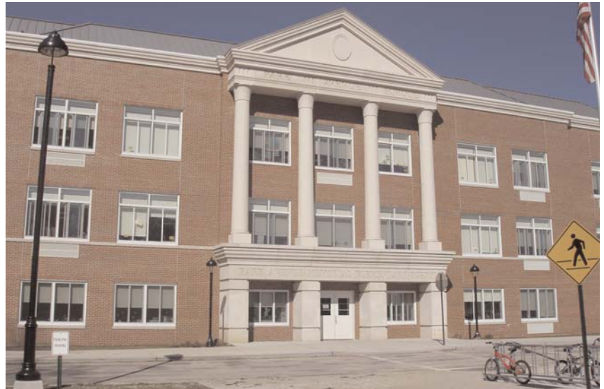
→ Amityville Park Avenue School Amityville, NY 120,000 sf school addition. Architect: LZA/Thornton Thomasetti
