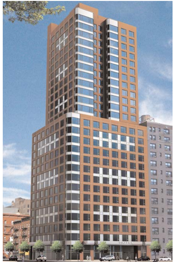
↑ Marriott Hotel 461 W. 34th Street New York, NY 28 story 300 key Marriott hotel with restaurants, meeting areas and various recreation and amenity areas. Total of approximately 200,000 sf. Architect: Karl Fischer Architect Owner: Atria Builders
